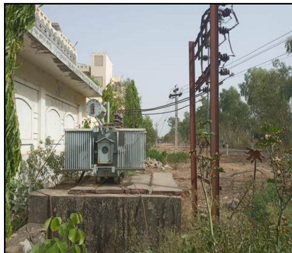
Figure 2.1:- 11 kV Feeder and 630 kVA and 500 kVA
